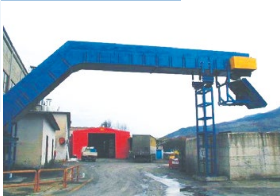
Heavy conveyor for scraps discharge
