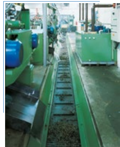
Hinged belt conveyor line
